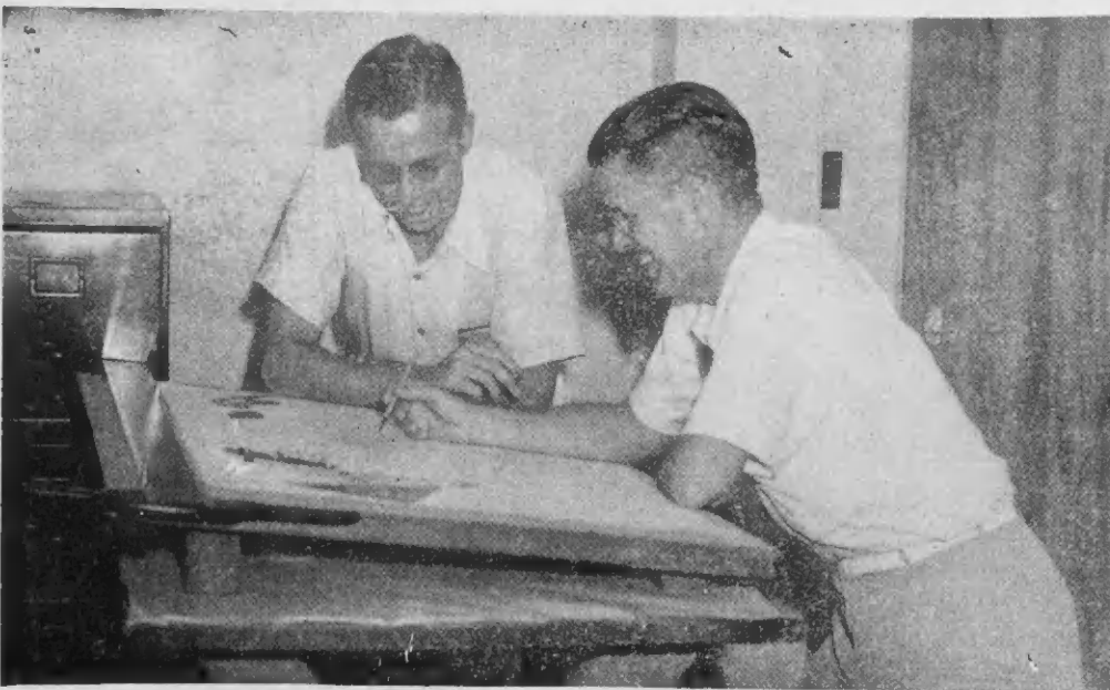
FRANK SHUFLIN, representative of the Robert Law Weed architectural firm of Florida, was a visitor last month. Shown above at right discussing preliminary plans with Colin Ward of Technical Service, he was here to consult on additional construction being planned at the Lago Sport Park, and on the design of a new Esso Club.
